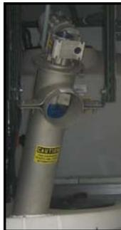
**Screening Unit** — The mechanical screening unit is used to separate and dewater non-organic solids before they enter the bioreactor. Proper screening is essential for MBR operation to prevent blocking of the feed space between the membrane envelopes.
