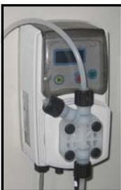
**Hypochlorite Injection** — A chemical injection system can be provided to inject sodium hypochlorite (bleach) into the CMBR filtrate to insure disinfection of the effluent. The hypochlorite injection system includes an injection pump and chemical day tank.
